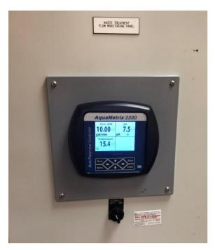
Mercy Hospital panel consisting of 1 AM-2300 Controller, pH, flow and temperature sensors.
